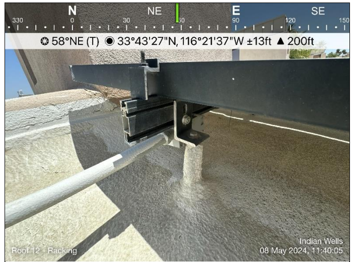
4. Connections are not torque marked
