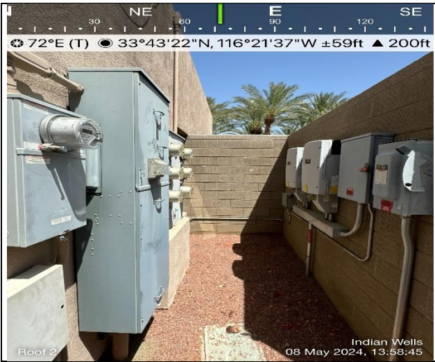
19. Roof 2 electrical corridor
