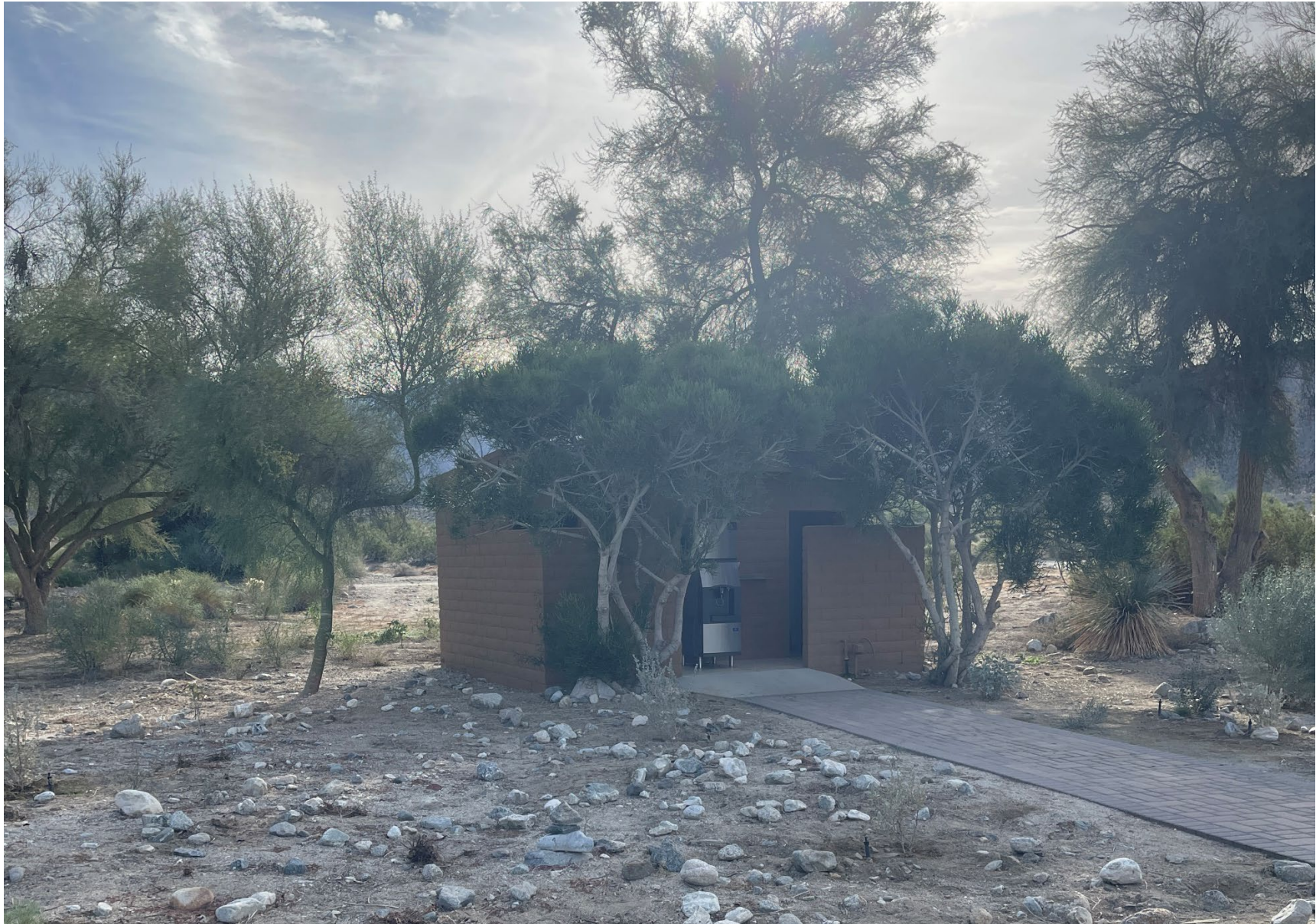
Existing Restrom to be Demolished
