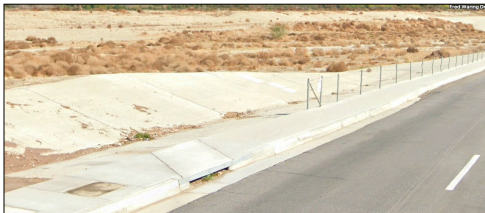
b) Sidepath and sidewalk at south end of river channel, facing east
