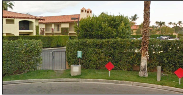
Figure 4-30: Indian Wells Lane north cul-de-sac – gate to Miramonte property
