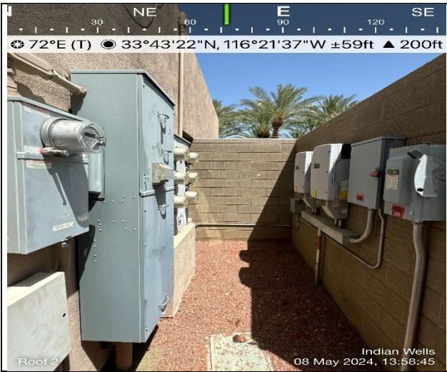
19. Roof 2 electrical corridor
