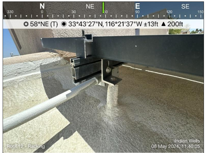
4. Connections are not torque marked
