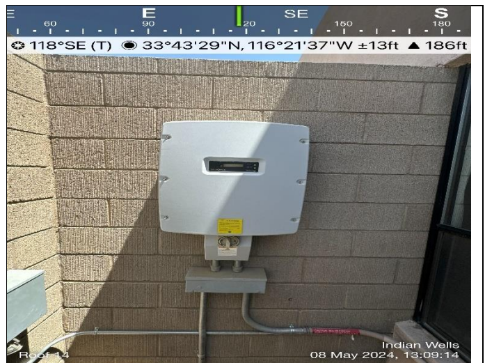
88. Roof 14 third inverter
