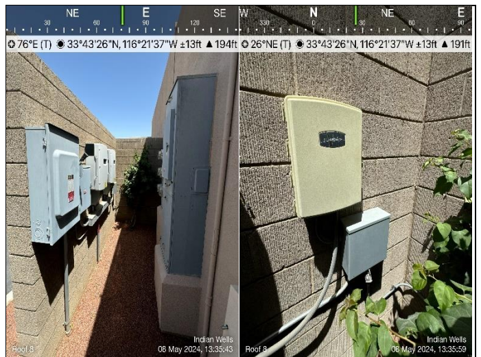
48. Roof 8 electrical corridor
