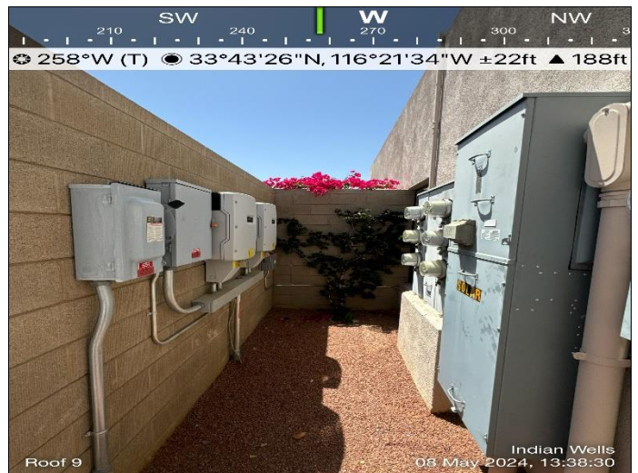
52. Roof 9 electrical corridor
