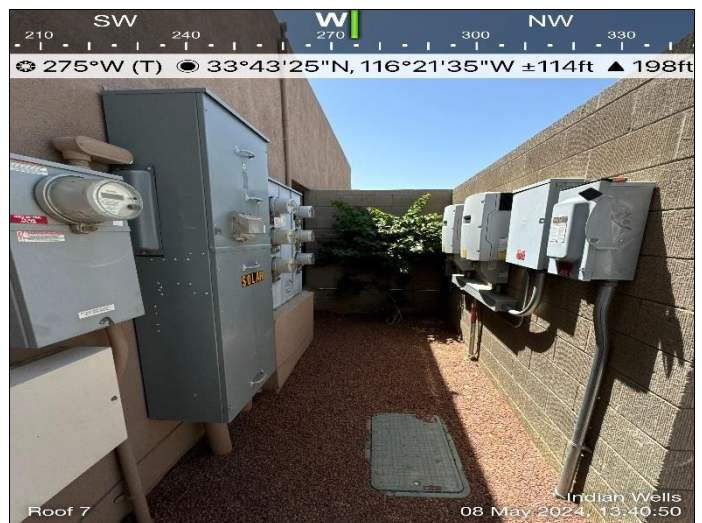
42. Roof 7 electrical corridor
