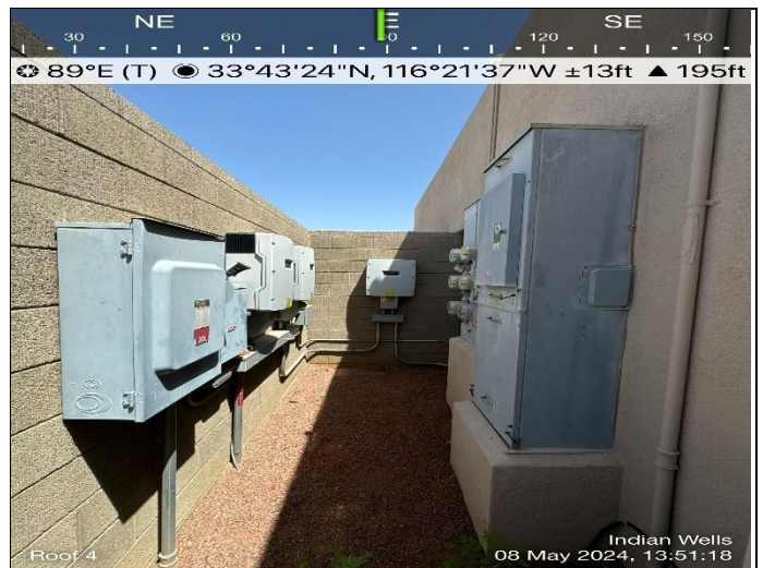
28. Roof 4 electrical corridor
