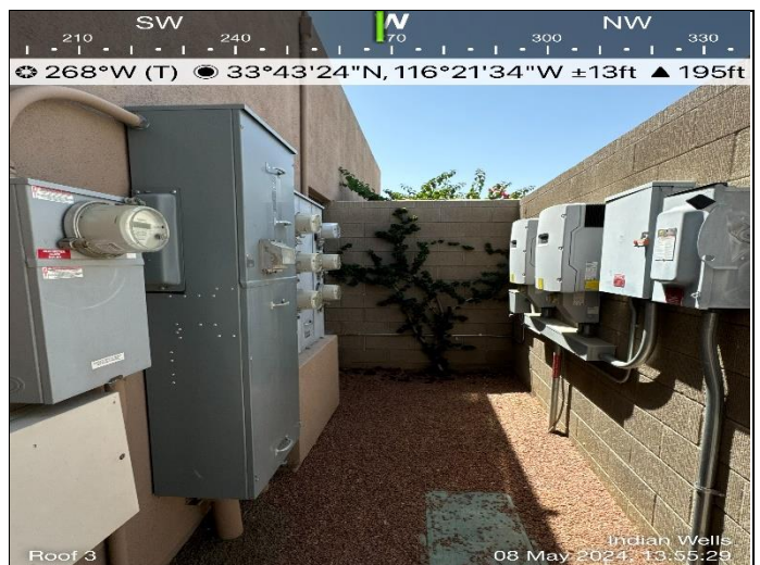
24. Roof 3 electrical corridor
